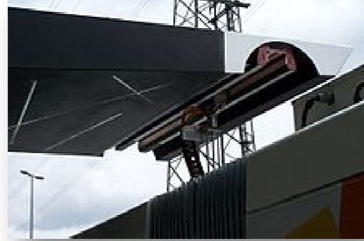
A battery electric bus charging station in Geneva, Switzerland
